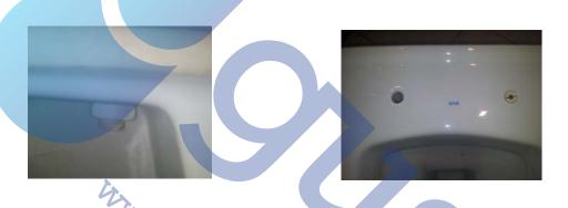
The top left picture shows the original Pluto fixing. This fixing is bolted in place at the time of manufacture. The top right picture shows the view from above.
